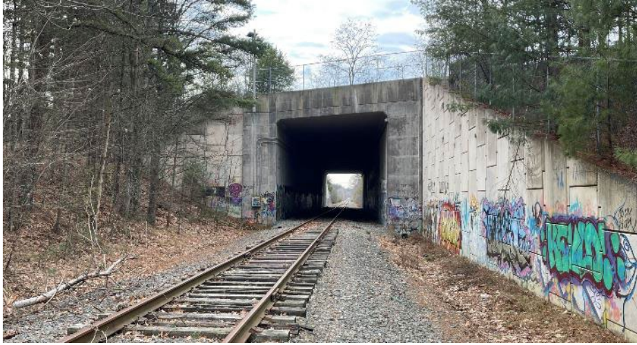
Route 196 – Topsham (Single Track Bridge)
