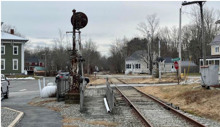
Weymouth Road – Richmond (Former Platform & Signal)
